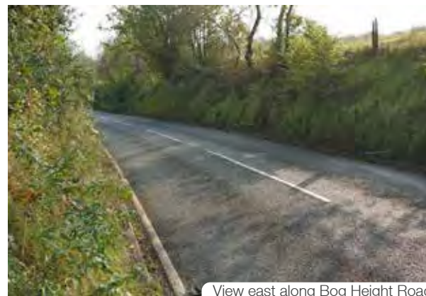
View east along Bog Height Road
