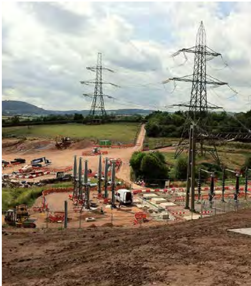
The undergrounding of electricity cables at Ross-on-Wye
