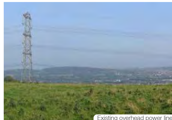
Existing overhead power lines
